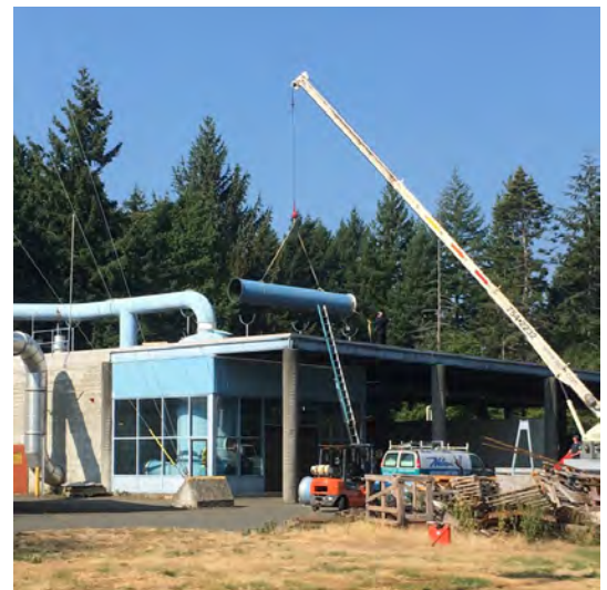
The existing air scrubber – which cleans the air of odour – undergoes a retrofit.
