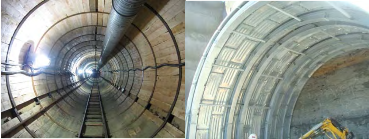
Figure 3: Example of steel ribs and lagging (left), and bolted liner plates (right)
