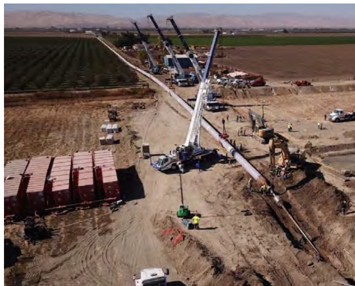
Figure 9- Example of product pipe layout for pullback into the reamed borehole.
