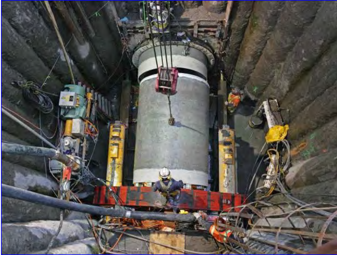
Figure 6 - Typical microtunnelling setup in jacking shaft. The direction of drive is to the top of the picture. The jacking equipment is the red and yellow frame surrounding the MTBM.
